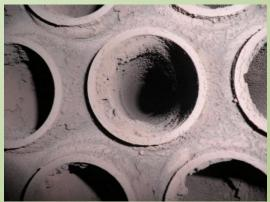
Due to low velocity of exhaust gas and poor atomization as well as combustion process, amount of deposits in smoke tubes increases drastically.
