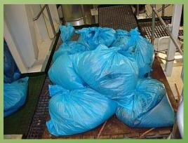
200-300 kg of deposits can be accumulated in smoke tubes over period of 4 months between washing (boiler's nominal steam output 1700kg/hr).
