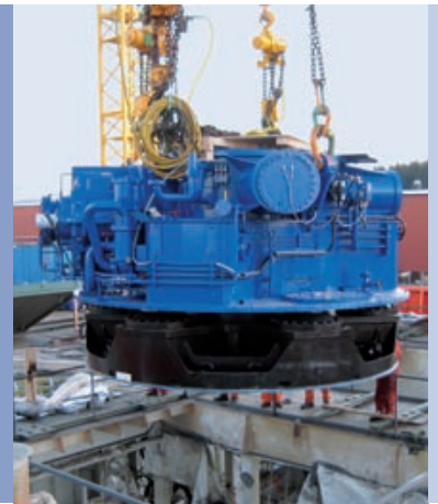
Preparations prior to installation
