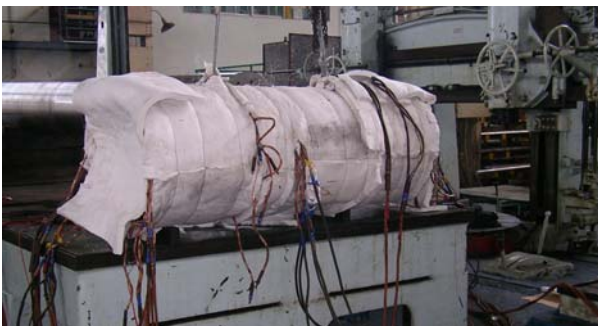
Figure 4. Liner heated for installation, horizontal.
