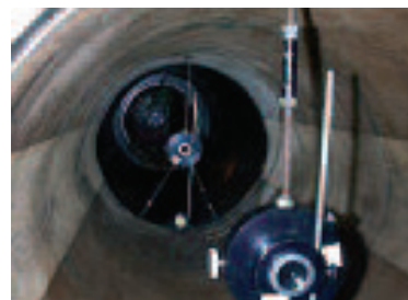
Optical sighting is one of four popular tried-and-tested methods used, either singly or together, to align shafts.
