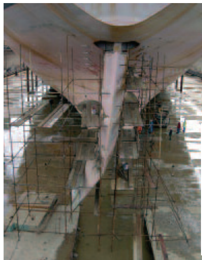
After the grounding of the Keymar in heavy weather, its owners engaged Lloyd's Register to check the vessels shaft alignment during each of the major stages of the vessels's repair
